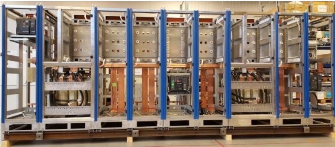
*Yaskawa multi-megawatt The Switch DC-Hub with electronic bus link to be fitted to Teekay tankers*
